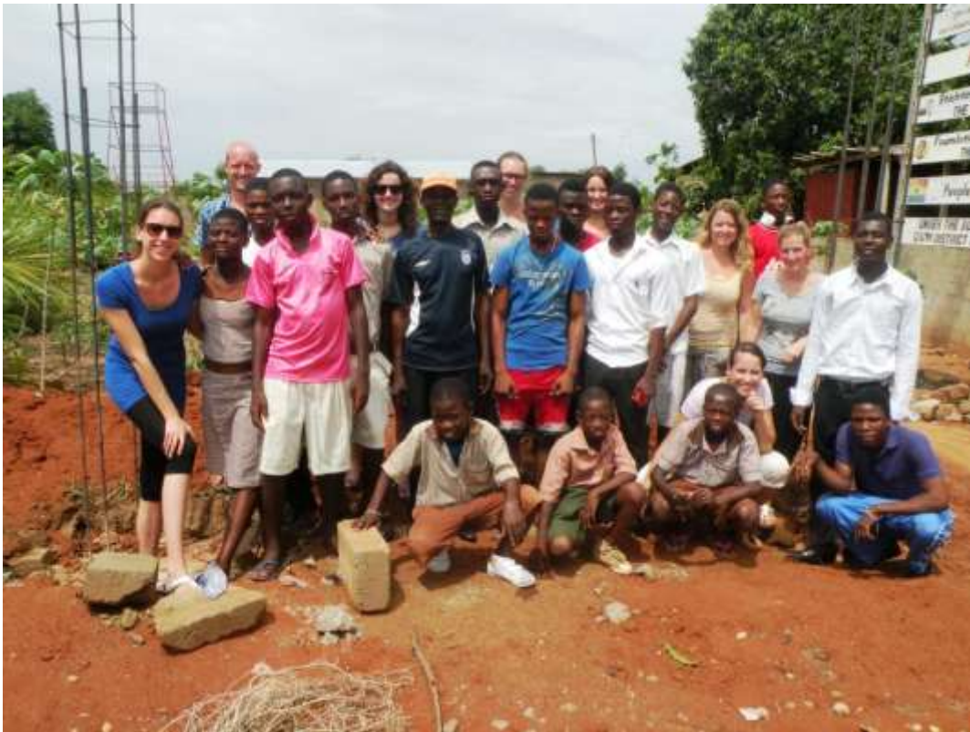
The project manager (middle with the orange cap) and some children of the Children’s Home, Let’s go Ghana’s programme manager Noor (left), current volunteers and interns in front of the (not yet finished) new children’s home building.
